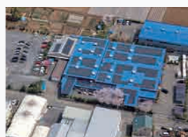
Factory rooftop, SHINANO INC.
